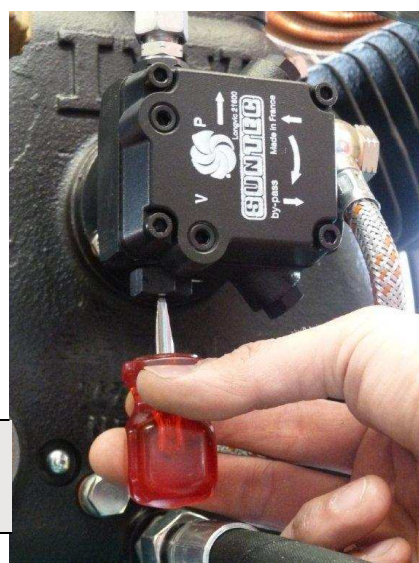
Adjusting the oil pressure
