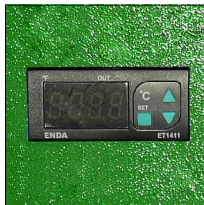
Oil Pressure Monitoring
